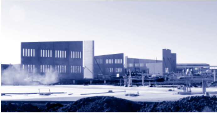
Construction of the new Wellington Correction Centre.
